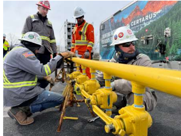
Prepare sampling header for fuel composition monitors
