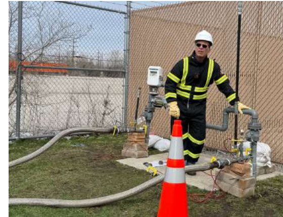
Connect to supply of natural gas and return of hydrogen blend to gas city
