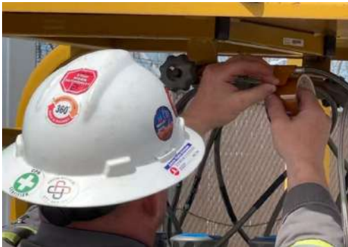
Leak test and apply hydrogen detection tape to joints
