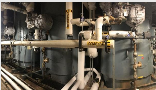
Existing steam-driven storage water heaters
